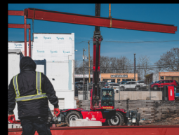
STEEL ERECTION
